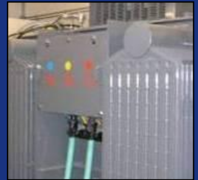
SF 6 insulated distribution transformers 2
